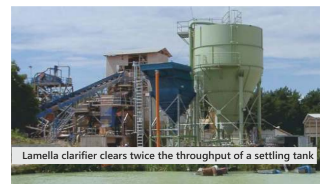
Waste water recycling for tunnelling
